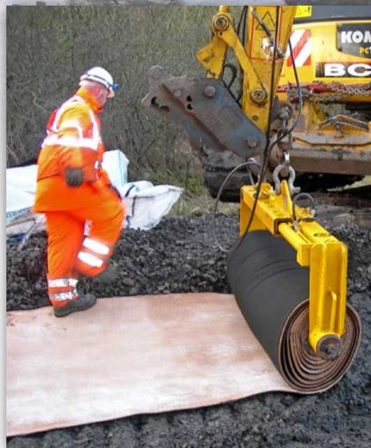
A roll of Geosand is installed using a roadtrailer.
