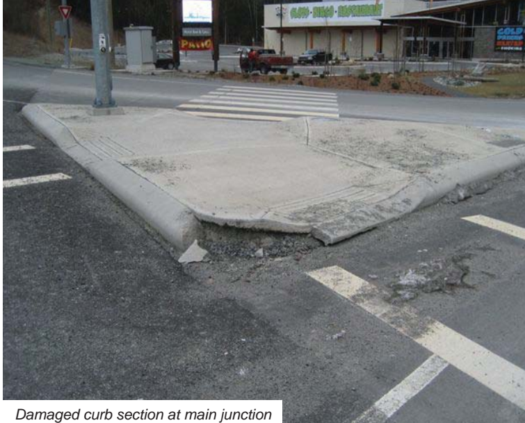
Damaged curb section at main junction
