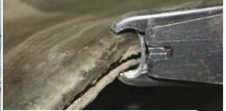
2 CC layers laid face to face and hog-ringed together
