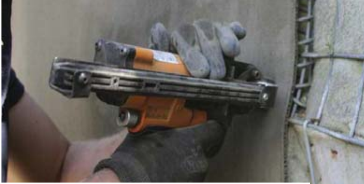
Pneumatic hog-ringer fixing CC to a gabion basket
